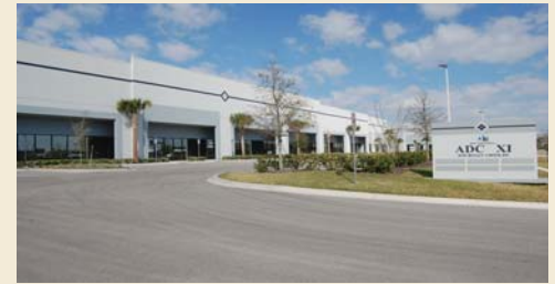
8429 Boggy Creek Road, Orlando, FL Lease
